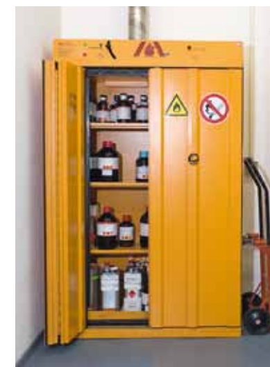
Safety cabinet for flammable liquids
