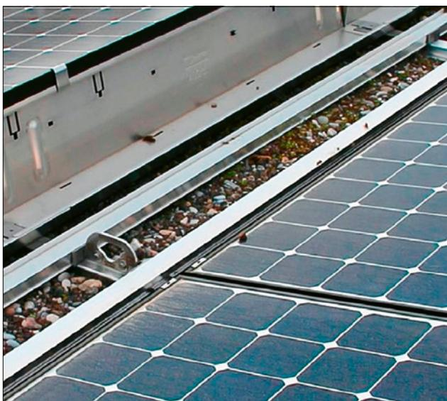
Anchor points for photovoltaic installations
