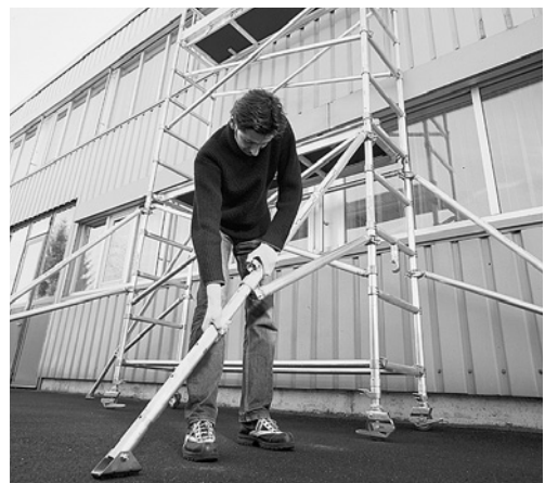
3 The assembly instructions specify the height from which supports must be fitted.
