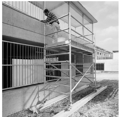
2 A firm foundation prevents the castors from sinking in without warning.
