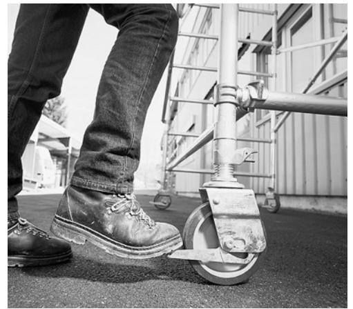
4 Castors must be secured to prevent the mobile scaffold tower from accidentally starting to roll.
