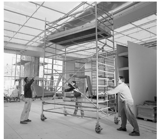
5 Mobile scaffold towers must never be moved when people are on them.
