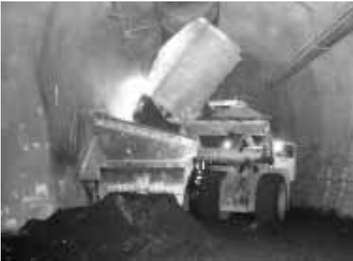
Fig. 3: Tyred-wheel loader during dumping. When choosing a PFS, the rough conditions to which the machines are subject must be considered.
